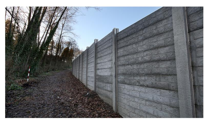
Natural Art Sound Wall utilizes the Canus Molding System to create a lightweight, and easy-to-install engineered product that maximizes sound reduction of environmental and ambient noise.
